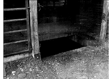
Access to manure pit where two died after entering a manure pit, Iowa FACE 2005 IA 024, 025.
