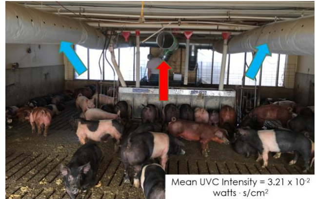
Figure 3. Untreated swine room air was drawn into the system (i.e., red arrow) with and treated UVC and MERV 16 filtration and returned to the room (i.e., blue arrows).
